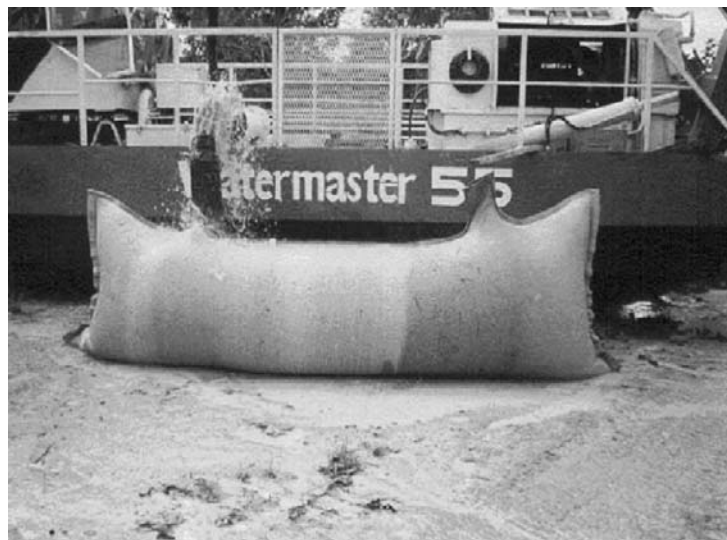
Gambar 2.12 Proses Pengisian Tube L = 10 meter , Malaysia 2000.
