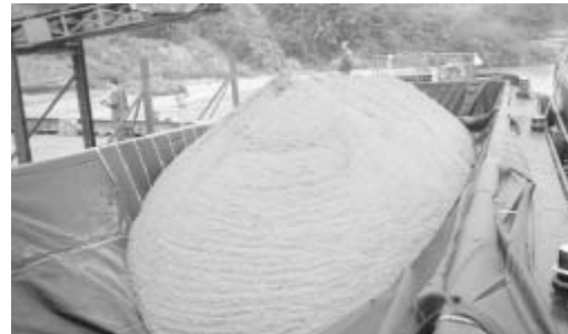
Gambar 2.7 Material pengisi geotube ( a ) Lumpur – lanau ( b ) Pasir
