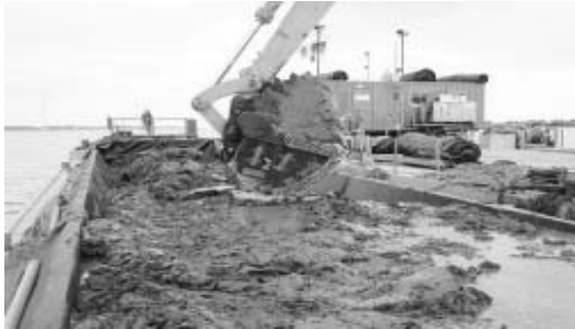
Gambar 2.7 Material pengisi geotube ( a ) Lumpur – lanau ( b ) Pasir
