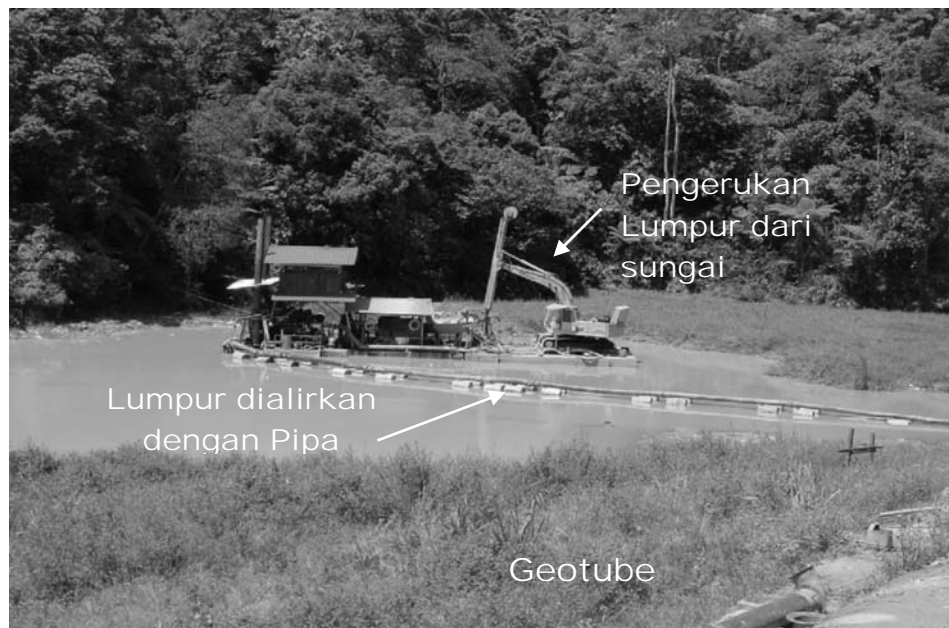
Gambar 2.15 Instalasi Geotube Cameron Highland, Malaysia.
